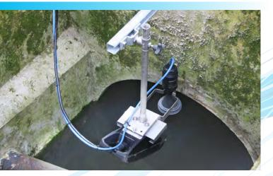
Non-contact RADAR flow measuring system
